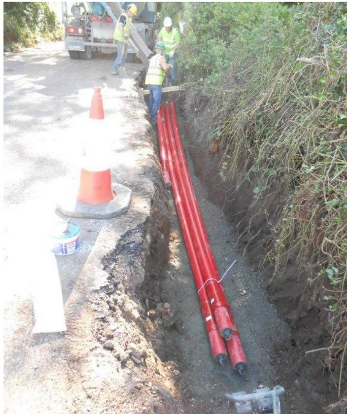
**Figure 3-10: Cable Duct Laying in Trefoil Configuration**
